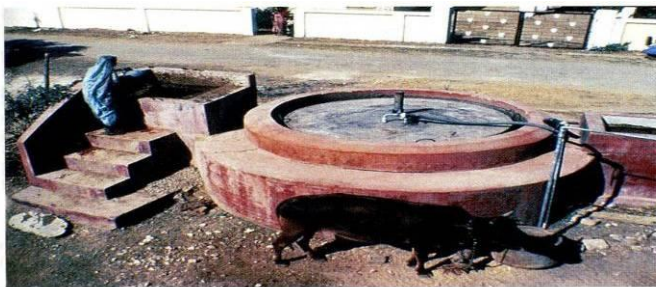
▲ FIGURE 15-22 Biogas power. Animal wastes are introduced to this unit in rural India and mixed with water. The wastes then decompose under anaerobic conditions, producing biogas.
